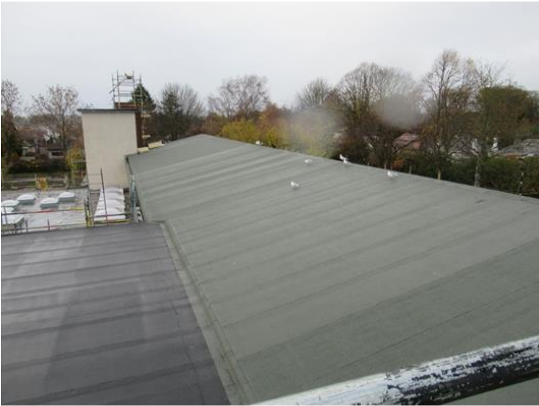
Photograph of Clermiston PS roof after enhancements
