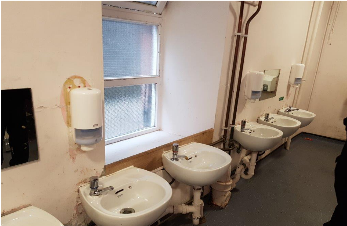
Photograph of Leith PS Infants Toilets before enhancements
