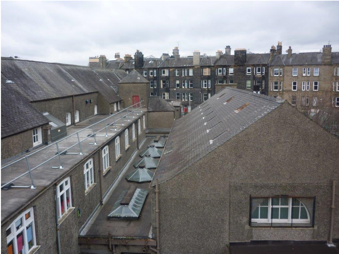
Photograph of St. Marys PS Roof before enhancements
